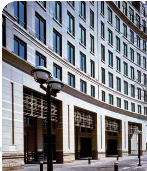
| EMA building in London
